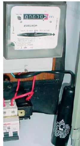
**Fig. 6:** HomeCap installation in the metering cabinet
